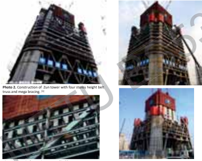
Photo 3. Detail of mega bracing profile. [1]
